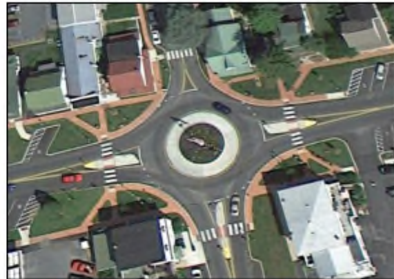
(Source: PennDOT Local Technical Assistance Program)
