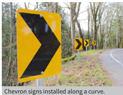
Chevron signs installed along a curve.
