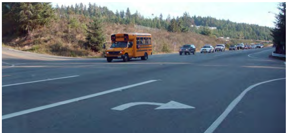
Example of a right-turn lane.
